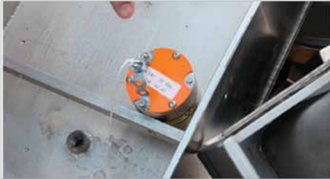
Ci Am-241 source in Tungsten shielding container
